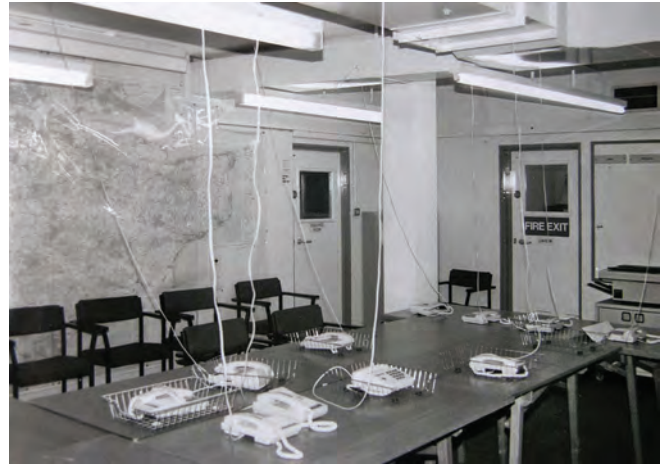
Control Room in the county control at Maidstone in 1988
